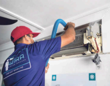
A technician with Wia Aircon Services, which has seen urgent requests for servicing increases by 40 per cent in the past three weekends, also has undertaken more extensive work such as changing air-con pipes and condensers almost daily.
